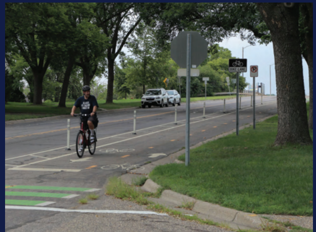
▲ Pelham Blvd: Delineators
