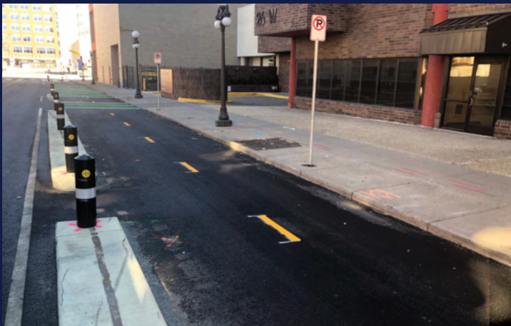
▲ 10th St downtown: Form-in-place curbs, bollards
